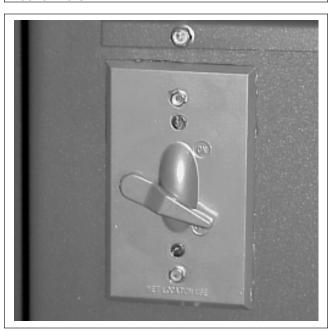
Figure 16. Heater's ON/OFF switch in OFF position.
